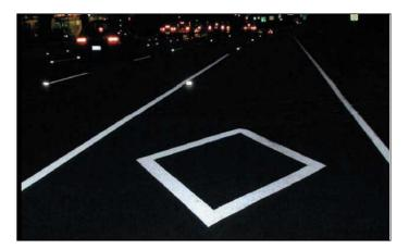
Figure 40 - Retro-Reflective Pavement Markings
